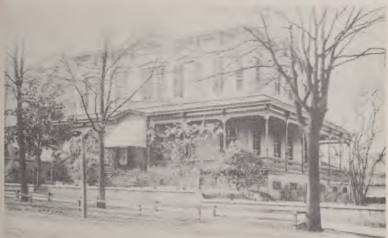
Semple-Knox-Saffold-Lehman-Goetter-LeGrand home at the SW corner of Court and Clayton Streets built about 1852 has been demolished.
